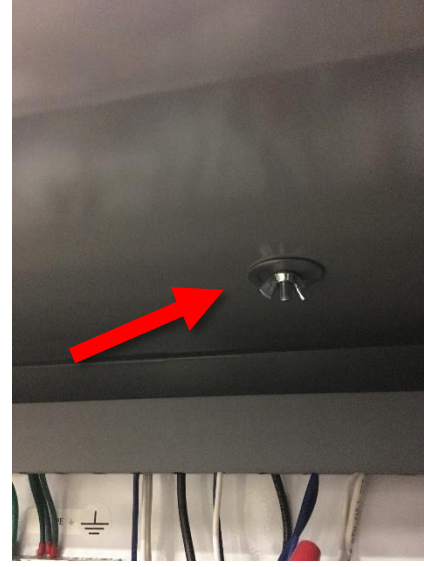
Figure 9. Figure showing the location of the electrical knockout on top of the electrical panel box. The knockout plug can be removed via a wingnut accessed from the inside of the electrical panel box.
