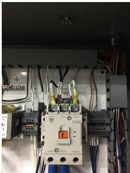
Figure 10. Primary contactor for Extrakt 110 and Extrakt 110+
