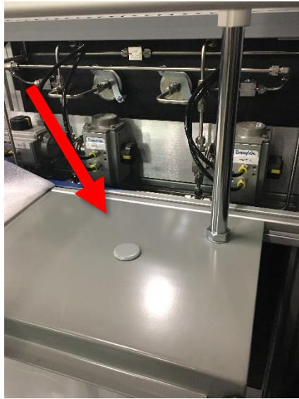
Figure 9. Figure showing the location of the electrical knockout on top of the electrical panel box. The knockout plug can be removed via a wingnut accessed from the inside of the electrical panel box.
