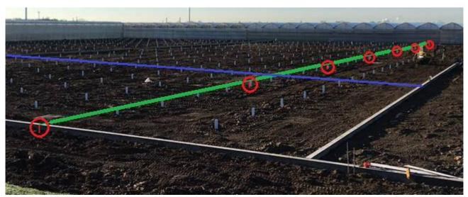
The red marks on the sketch above are the steel pins. The green line is the wire tightened to the pins. A second line (blue) is placed to determine the exact location of the foundation posts.
