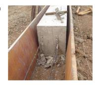
After the concrete is poured, a compactor is used to compact the concrete by vibrating quickly. After the concrete is settled, the workers flatten out the top of the wall with plasterwork tools, for a smooth finish. It is very important this is done by a specialized worker. In a later stage a profile has to be drilled onto the wall for the gable system If there is too
