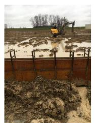
After the forming is placed, U brackets are installed to keep the forming in position. These brackets have to be placed carefully by an experienced worker
