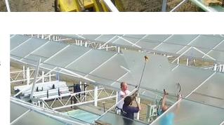
When a ventilation window has to be installed, another component is used. Instead of placing a whole piece of glass, the crew places the under vent window. A extra glazing bar is used about 1/3 of the plate of glass. A third glazing bar is put in place to keep the smaller window in position. The ventilation windows has a profile attached to it, this profile is designed to fit and to allow the windows from opening and closing.
