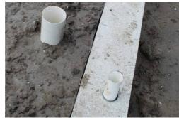
the wall has a gap, where a rainwater discharge tube fits perfectly.
