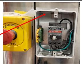
The first live wire is attached to the contactor section "1L1".
